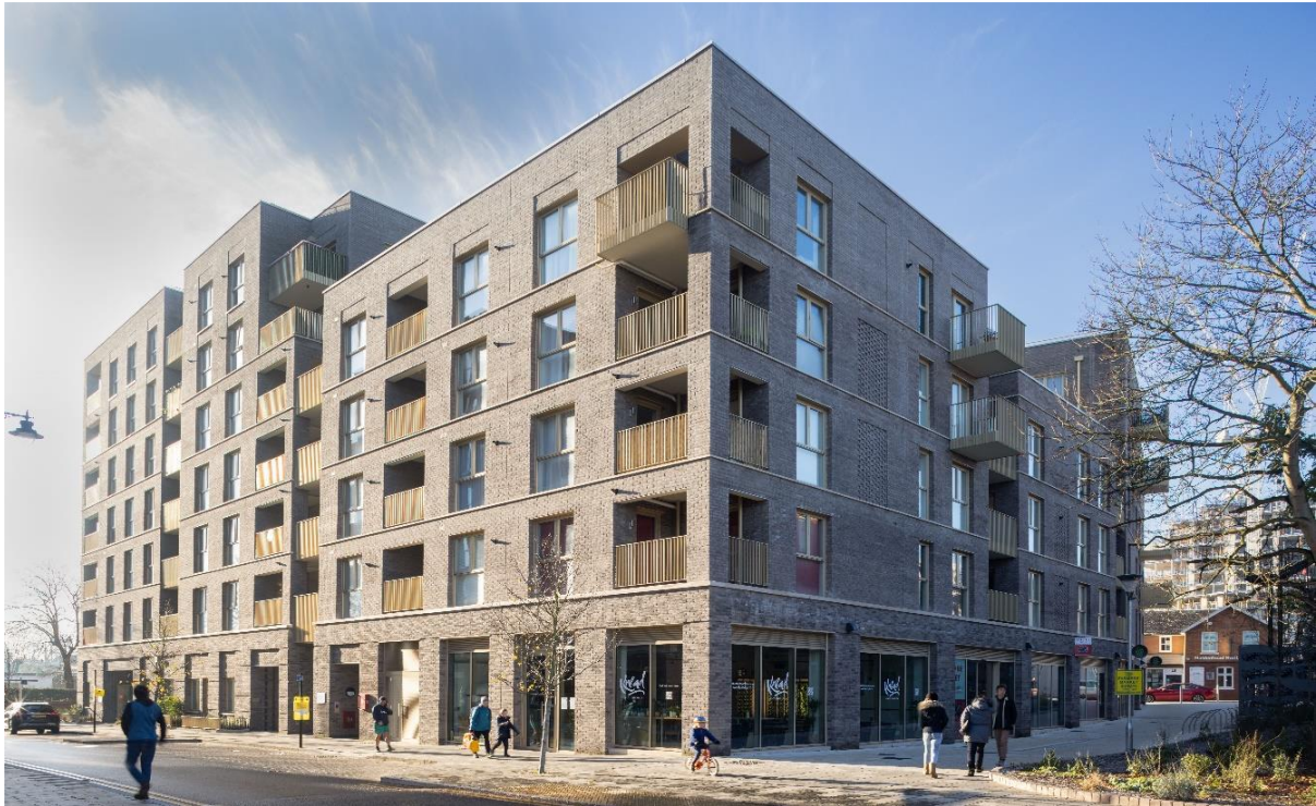
BLOCK D – TRINITY PLACE, YORK ROAD
